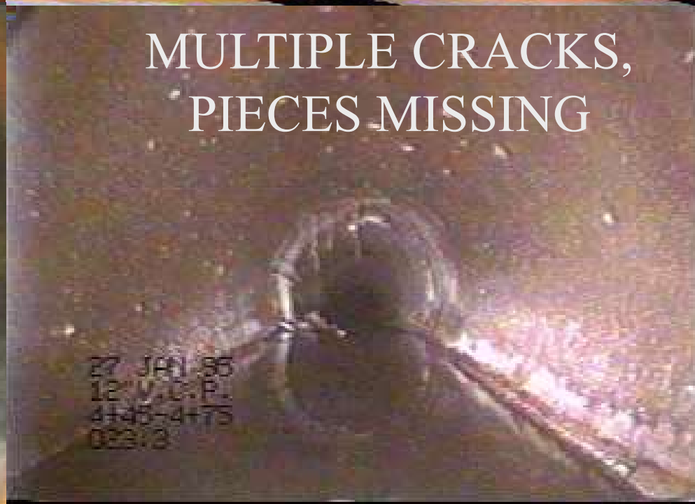
CRACKED OR CRUSHED PIPE
