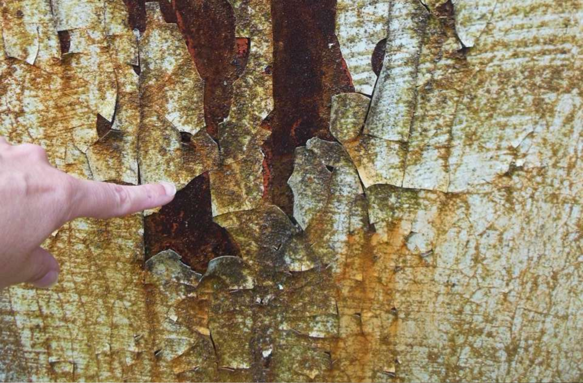
Coating Deterioration
