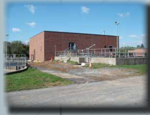
Biosolids Drying Facility
